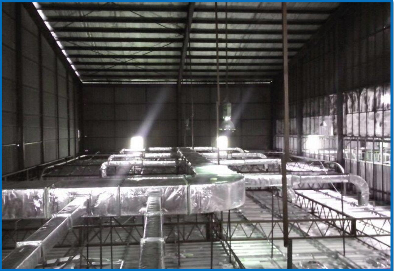
Ducting Work (Air-Conditioning Line) – Sungai Petani
