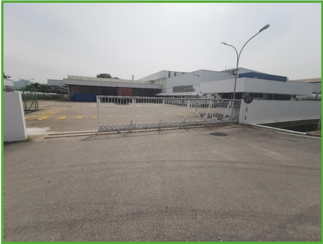
Construct Factory Building – Tikam Batu
