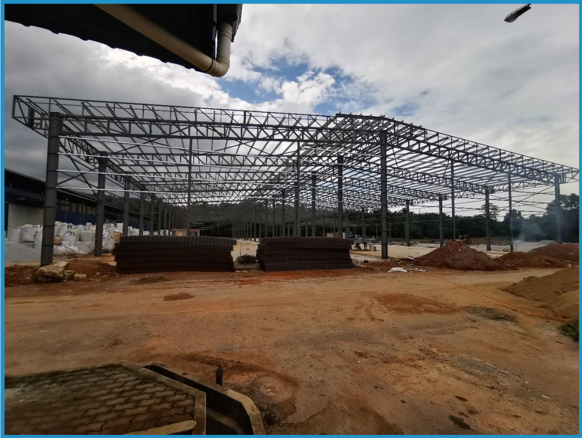
Roofing Super Structure
