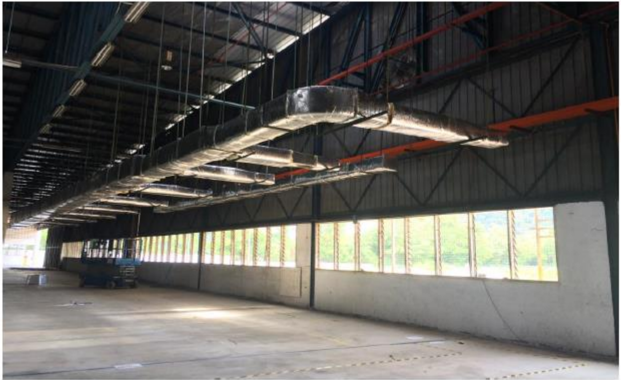
Air Cond Duct Work – Juru
