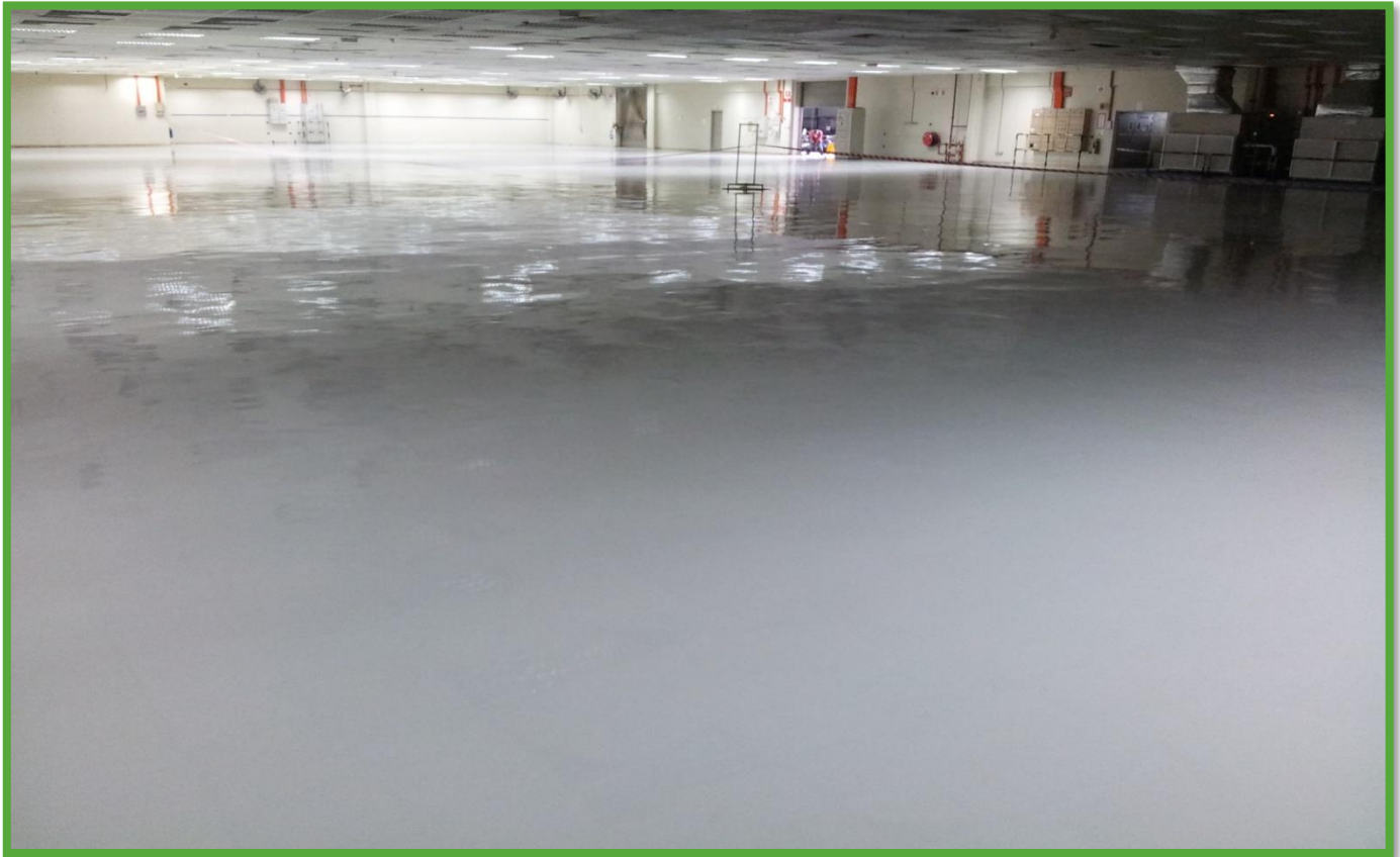
Waterproof & Heavy Duty Epoxy Floor – Prai
