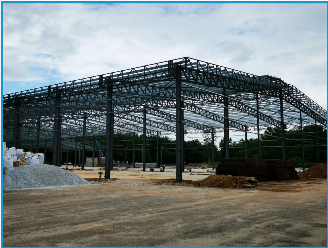
Roofing Truss Structure
