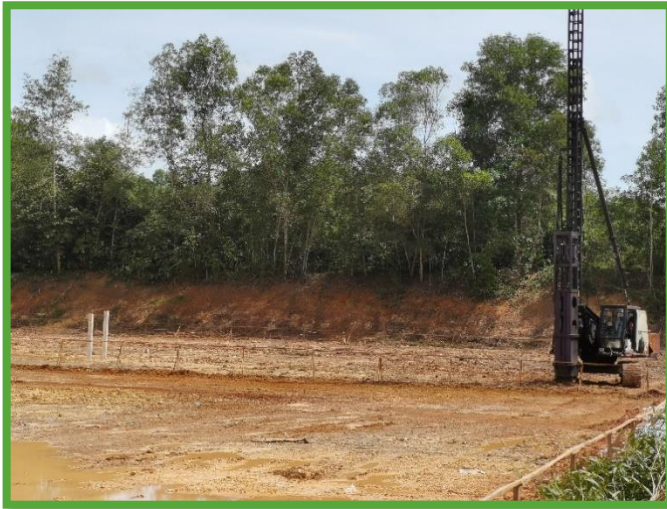
Piling – A frame
