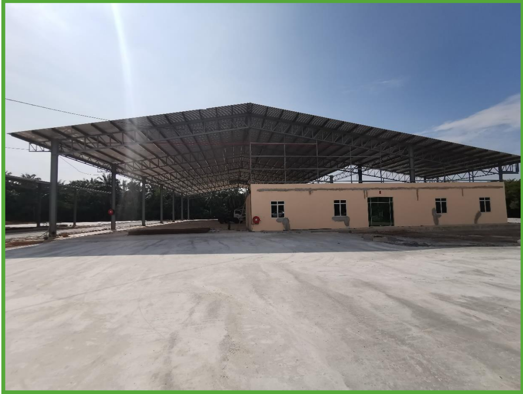
Construct Factory Building – Sungai Petani
