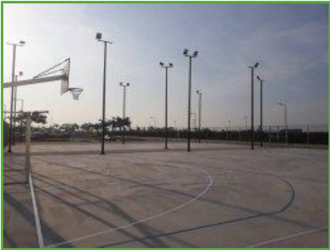
Construct Basketball Court – Batu Kawan
