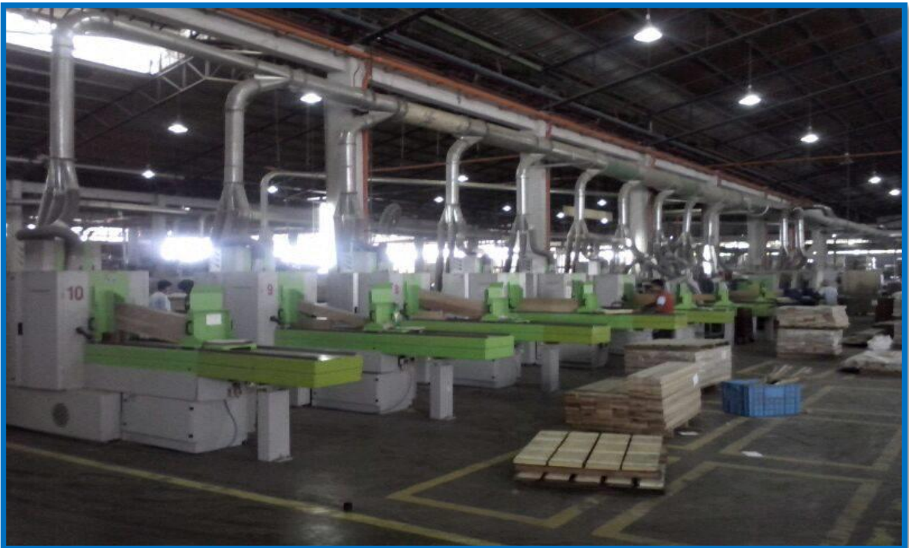
Exhaust Ducting Work – Sungai Petani
