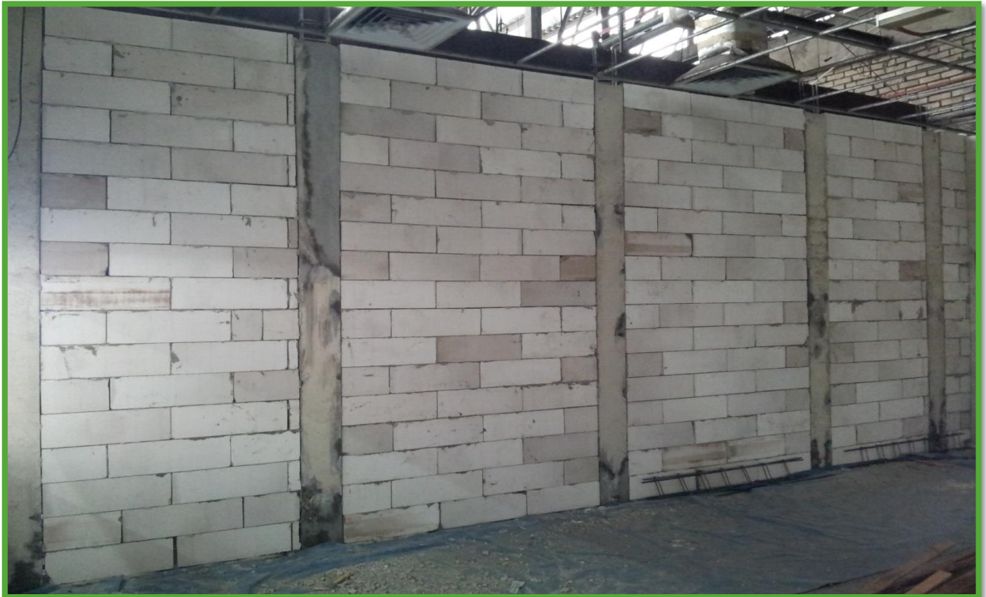
Two Hour Fire Rated Brick Wall – Prai
