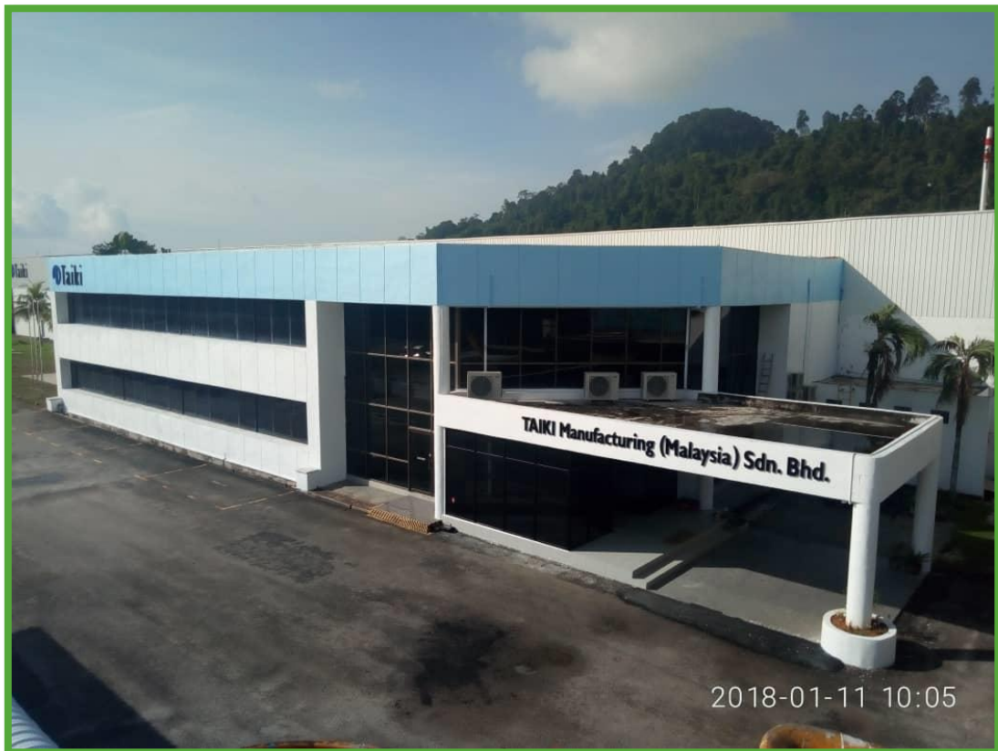
Construct Factory Building – Juru
